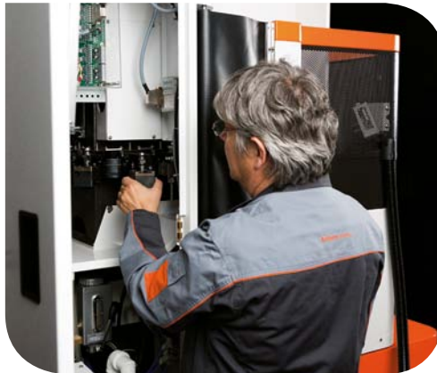
Manual loading location
